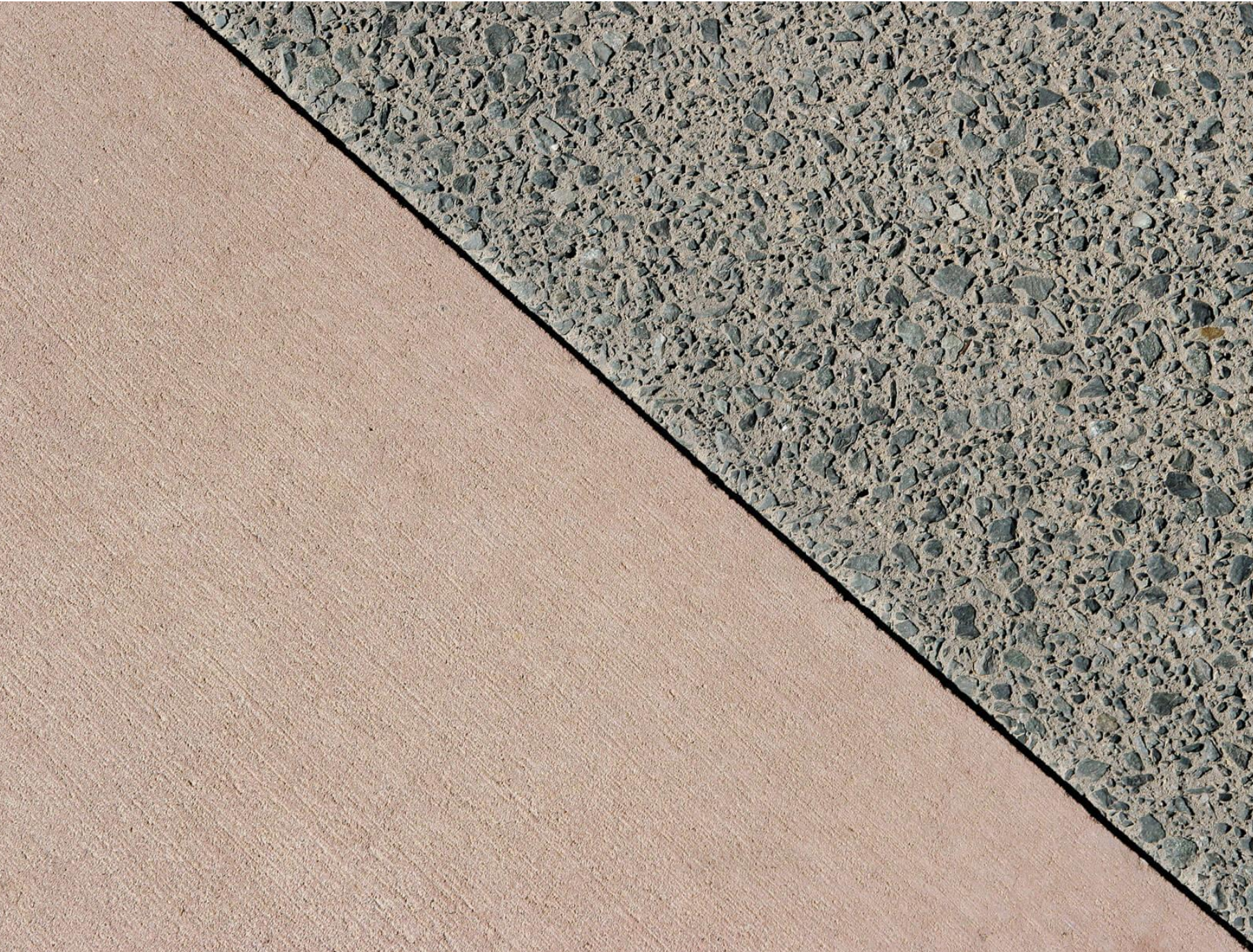
FEATURE COLOURED AND EXPOSED AGGREGATE CONCRETE AREAS
